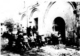
Fig. 14.15. The sarcophagus of Czarina Natalya Naryshkina taken away from the Voznesenskiy Nunnery in 1929. After the transportation of the female sarcophagi to the Arkhangelskiy Cathedral, the Voznesenskiy Nunnery was demolished. Taken from [107], page 245.
